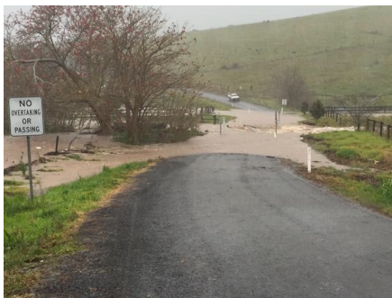
Flooded causeway on Mt Brandon Rd —>
