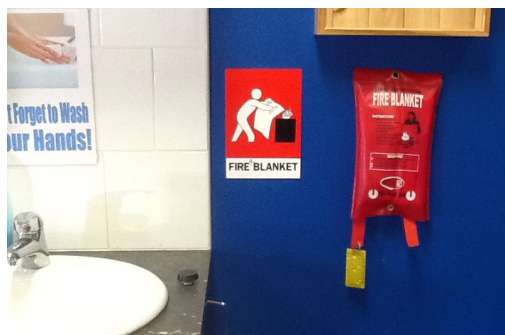
New Location of Fire Blanket
